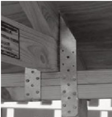
Roof to wall Connections
