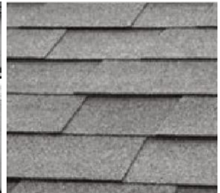
Upgrade of roof coverings
