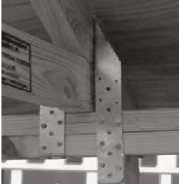
Example of Roof to wall Connections
