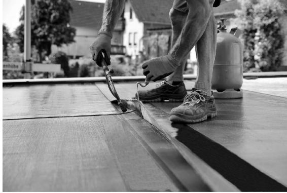
Exterior Secondary Water Barrier
