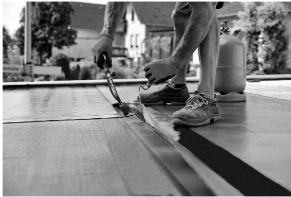
Exterior Secondary Water Barrier
