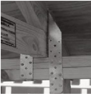
Roof to wall Connections
