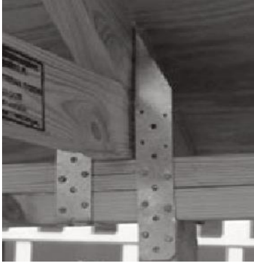
Example of Roof to wall Connections
