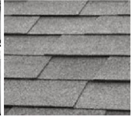
Example of Upgrade of roof coverings
